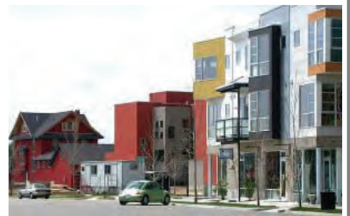
→ Prospect New Town in Longmont, CO has a mix of housing options
